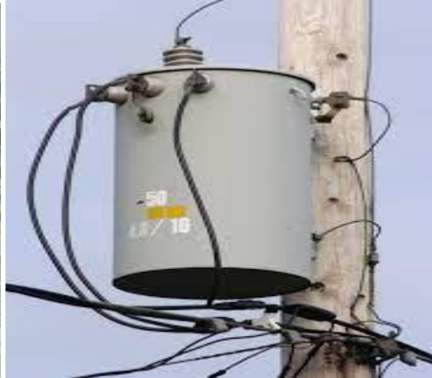
b) Step-down or distribution transformer.
